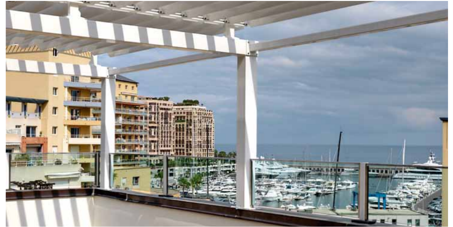
Baie Marquet, Cap d'Ail (France), 2012 - project by Longo Palmarini Architecture & Partners, photos courtesy of Andrea Martiradonna
